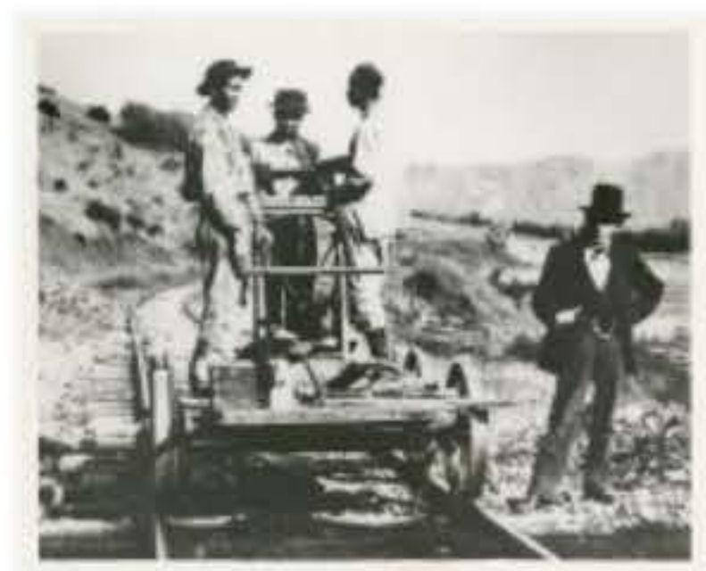
1876- Chinese laborers on a handcar during construction of Central Pacific Railroad line between Bakersfield & Los Angeles. This work (by Andrew J. Russell), identified by Oakland Museum of California , is free of known copyright restrictions.
